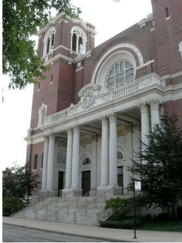
IL_Cook County_St Mary of the Angels Church001
