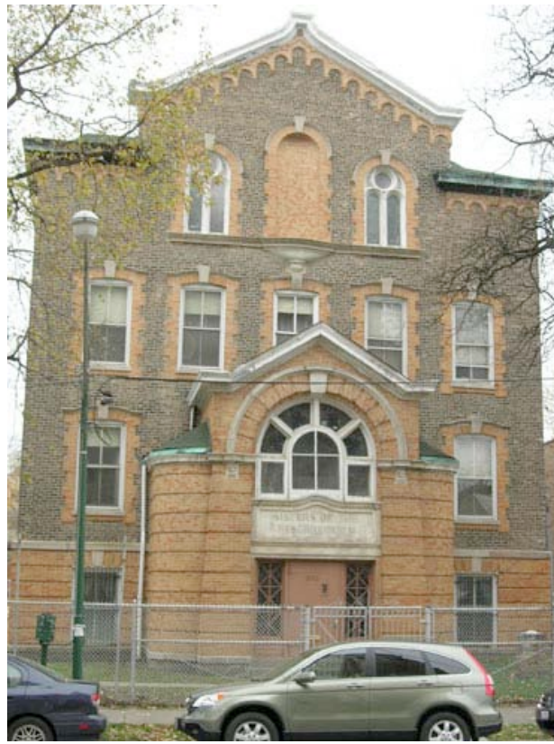
IL_Cook County_St Mary of the Angels Church008
