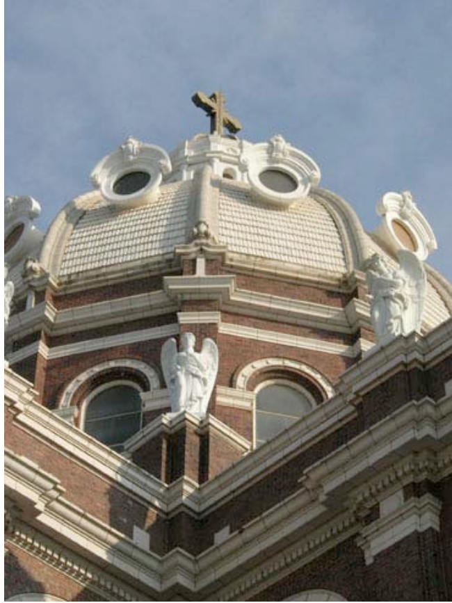
IL_Cook County_St Mary of the Angels Church005
