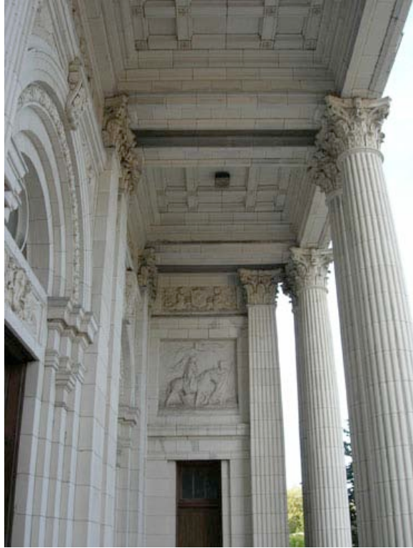
IL_Cook County_St Mary of the Angels Church007
