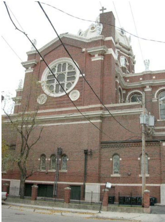
IL_Cook County_St Mary of the Angels Church004
