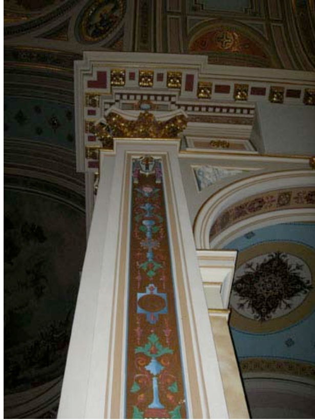
IL_Cook County_St Mary of the Angels Church015
