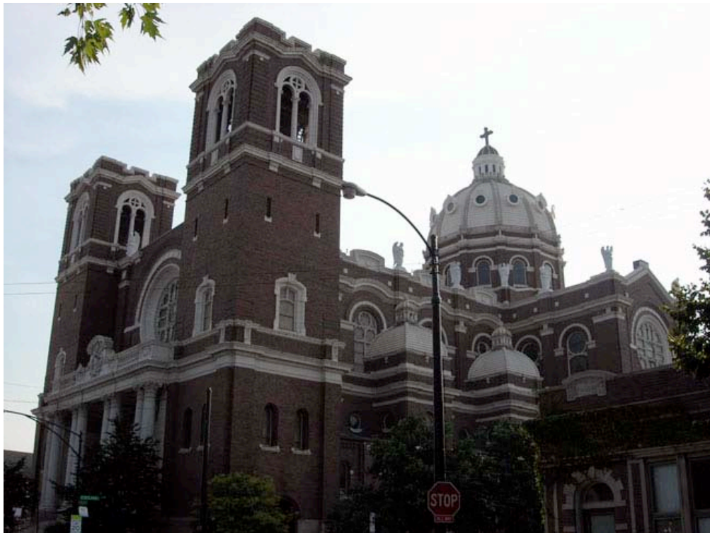
IL_Cook County_St Mary of the Angels Church002
