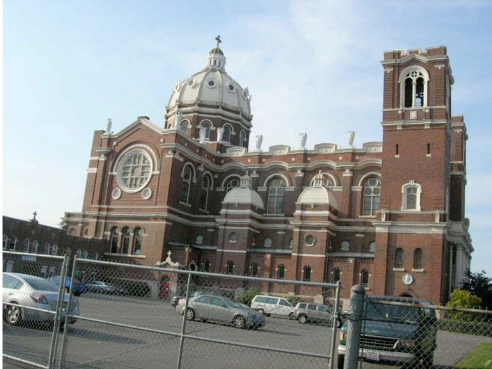
IL_Cook County_St Mary of the Angels Church003
