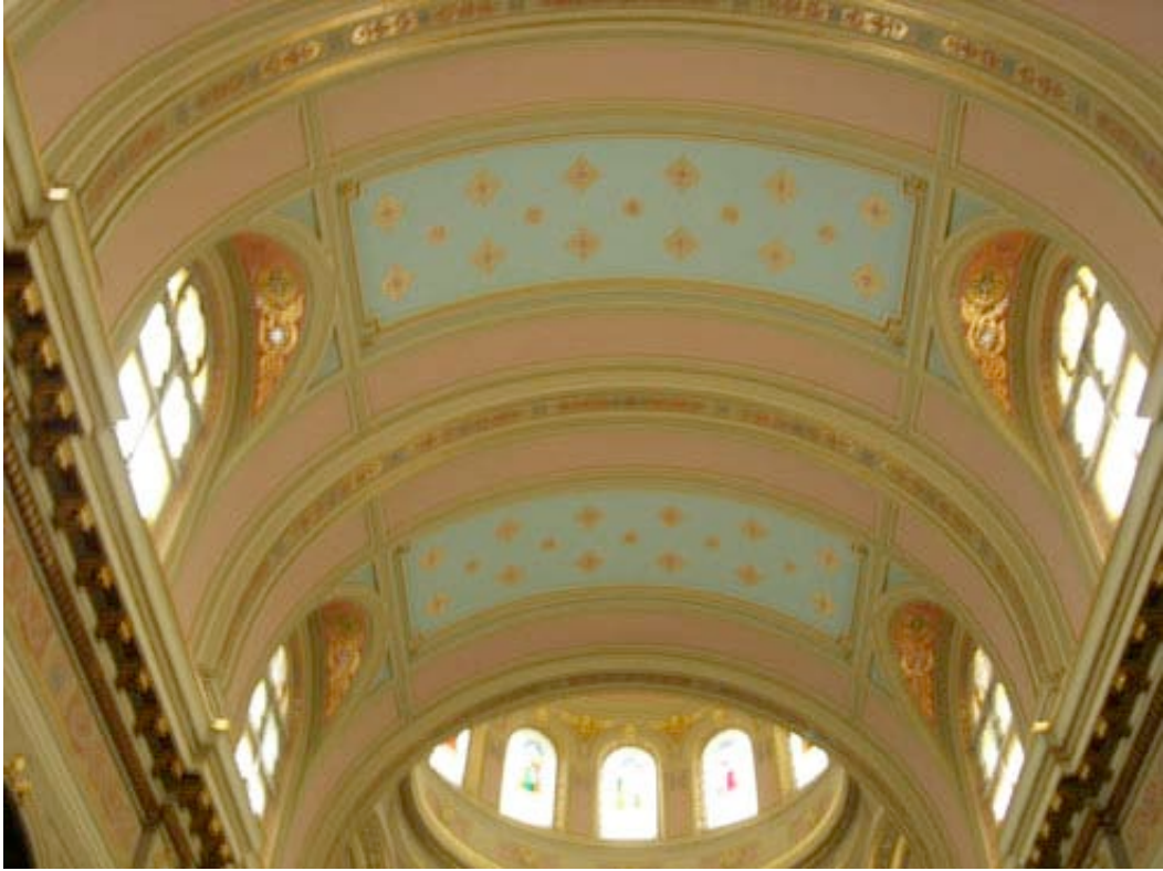
IL_Cook County_St Mary of the Angels Church013
