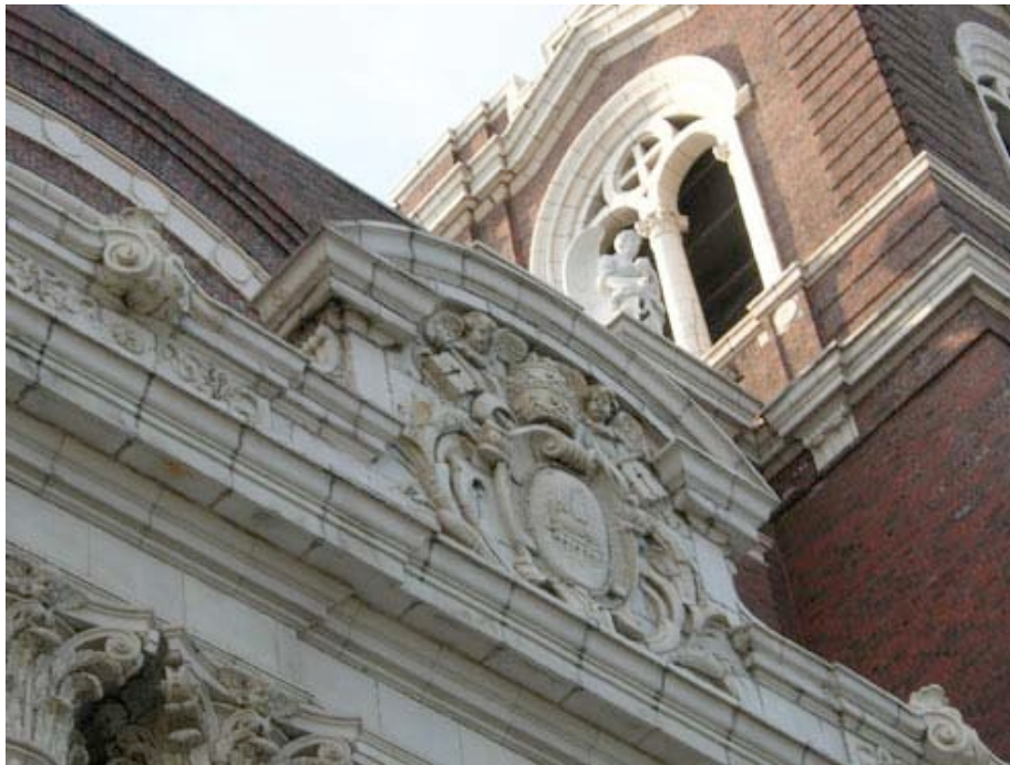
IL_Cook County_St Mary of the Angels Church006
