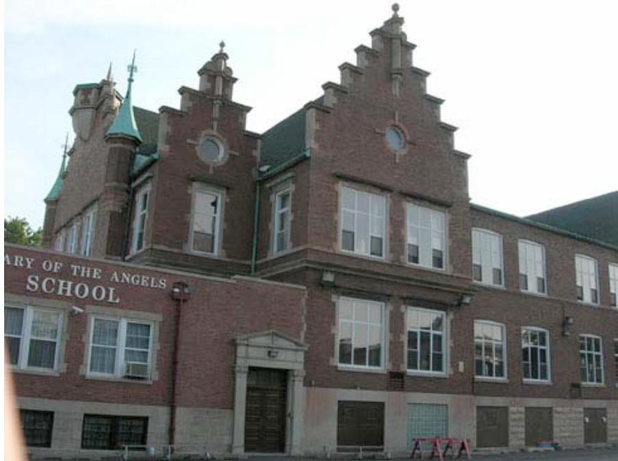
IL_Cook County_St Mary of the Angels Church009
